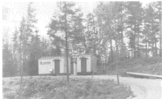
Pictured top is Bell Telephone dial exchange at Mine Centre. Below is Bear Passage dial exchange. Located east on Highway Eleven, the stations were built simultaneous with the highway; one in what was once a roaring mining town; the other in solid bush.
