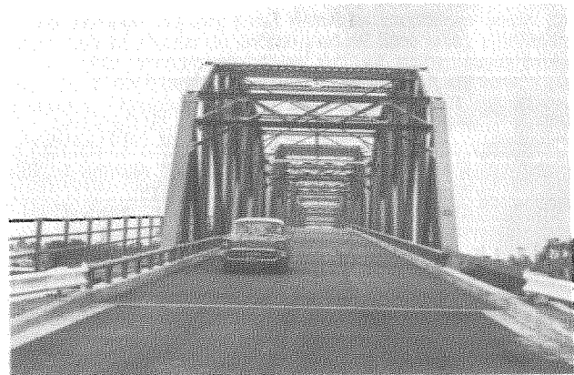
International bridge connecting Baudette on Minnesota Highway No. 11 with Rainy River on western terminus of Toronto to Rainy River, Ontario Highway No. 11. Note unique anti-snow Bridge decking. A Barnett-McQueen (Fort William) bridge structure.
