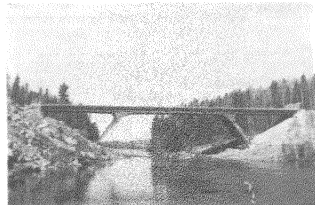
The Crilly bridge across Seine River, is a unique structure in that because of its A-frame design it requires much less steel than normally would be required to span an equivalent distance. Erected by Barnett-McQueen, Fort William. Marvellous fishing here. Majestic scenery. — photo by A. J. Klaus
