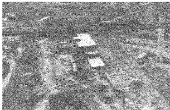
PROCESSING AND PELLETIZING PLANT NOW UNDER CONSTRUCTION
