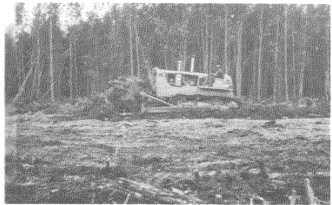
Roughing out right-of-way and road bed
