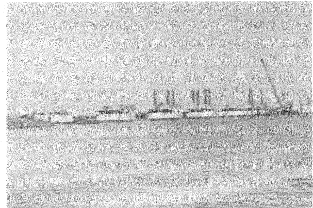
West End of Causeway High Level Bridge structure under construction.
