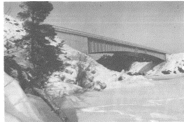
Bear Passage bridge 25 miles east of Fort Frances, spans Rainy Lake. It was a 1964 design award winner, featuring longest welded plate girder span built in Canada. The 491-foot bridge, including pouring of 1700 cubic yards of concrete counter balances is unique in Canada in that no piers could be erected to support the bridge structure. Erected under adverse conditions in middle of winter, to hasten highway construction, by Barnett-McQueen, Fort William. Magnificent scenic views.
