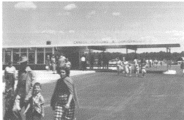
Customs Building at Rainy River Bridge.
