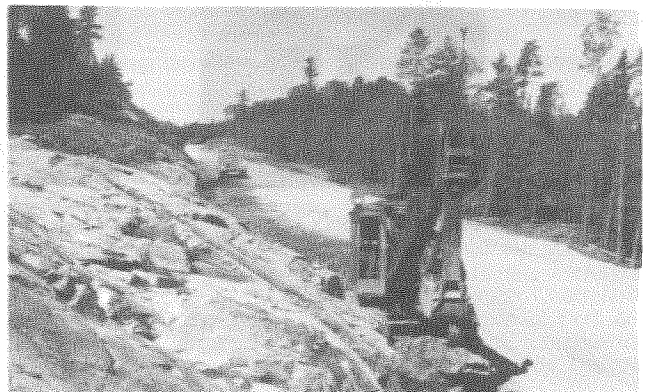
Dressing shoulders and cleaning roadside ditches
